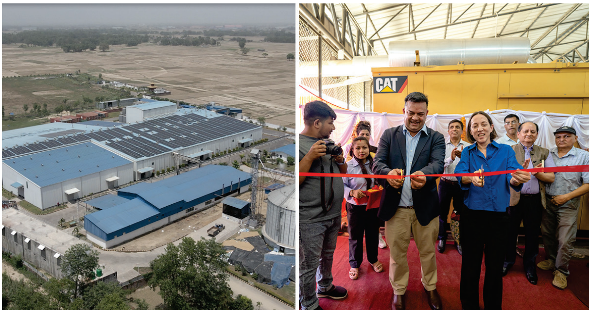
(Left) The 500kW rooftop solar installation at Raj Brewery, Nawalparasi. (Right) Raj Brewery Managing Director, Raj Bahadur Shah and InfraCo Asia CEO, Claudine Lim cut the ribbon at the system's inverter room.
